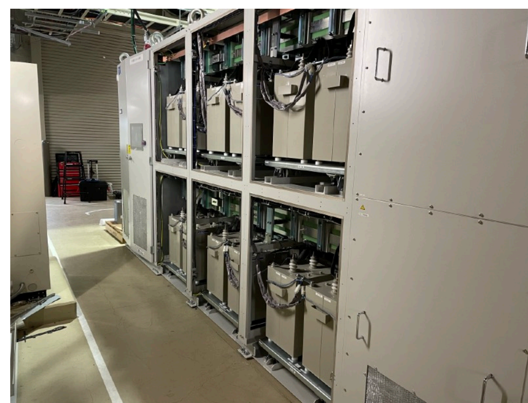
3rd PS and new capacitors installed
