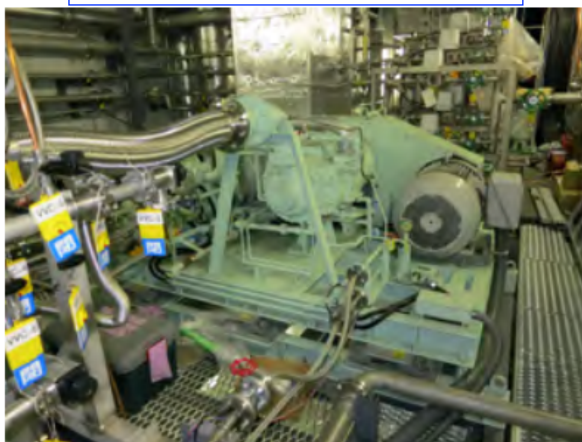
Existing He compressor for target
