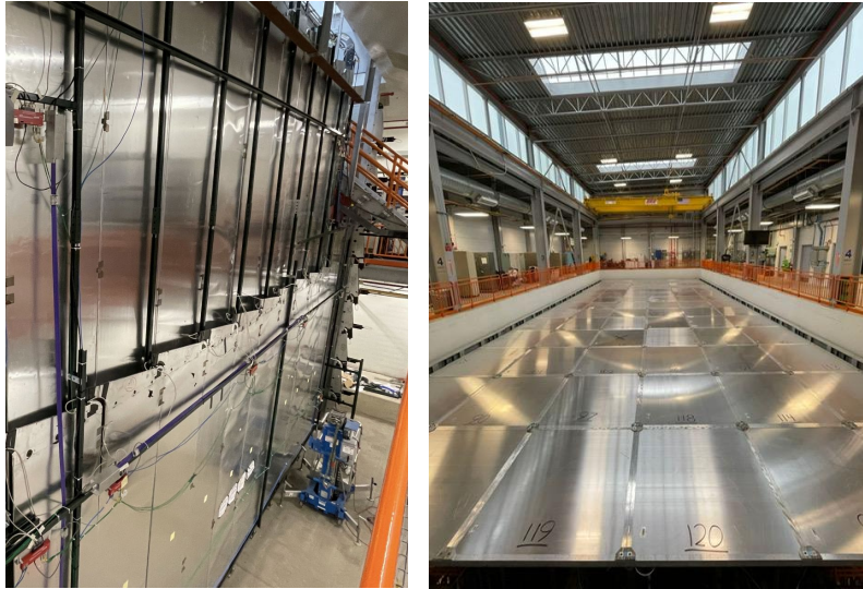
Side and Top CRT modules installed surrounding the ICARUS Cryostat.
