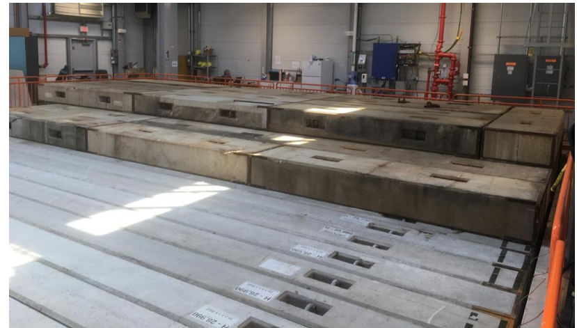
Second (of 3) concrete layers being installed above the ICARUS top CRT level.
