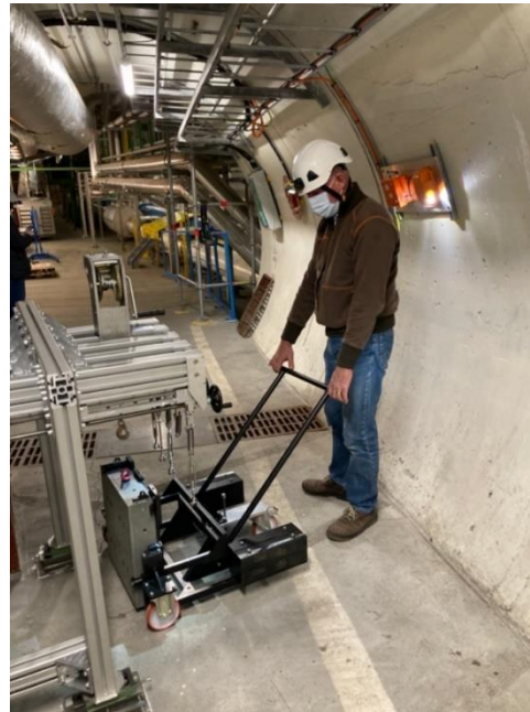
Trolley carrying ECC Brick
