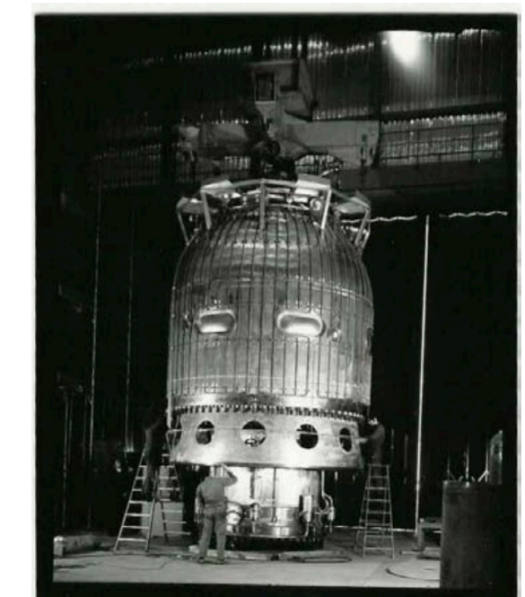
Fig. 7. The Big European Bubble Chamber (BEBC): the 3.7 m liquid container is shown at the top of the left figure, while it is being lowered into place; the right picture shows the body and in particular the expansion piston at the bottom. On the left, BEBC is shown with the external muon identifier composed of a set of electronic detectors. The superconducting coil is before the electronic detectors. BEBC, filled with H 2 , D 2 or H/Neon was used mainly with neutrino beams.
